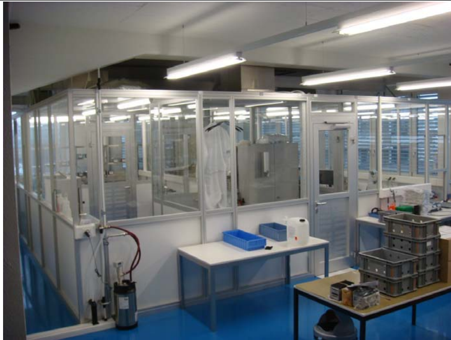
Image 1: Clean room from outside
