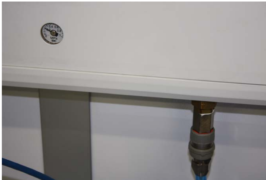
Image 14: Distributionsystem for compressed air
